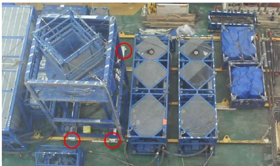
Figure 1 General View on Sand Silo location
