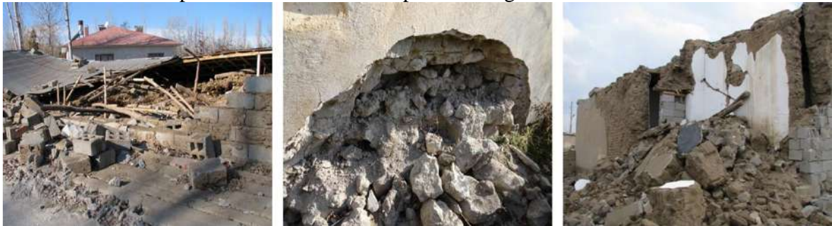
Figure 1. Out-of-plane behavior due to use of poor-quality masonry material
