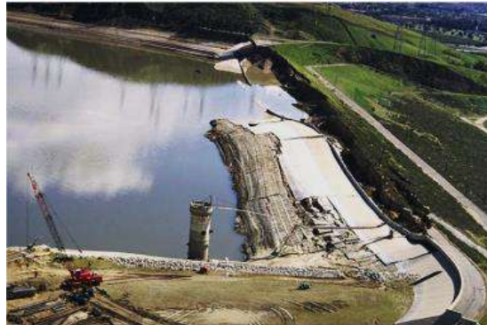
Figure 3. Dam failure due to liquefaction of water-saturated soil [8]
