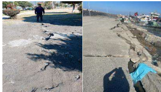
Figure 10. Surface manifestations of the sand boil as seismic liquefaction in Iskenderun Hatay (left), lateral spread due to liquefaction in the fishing harbor area in Iskenderun, Hatay (right) [19]
