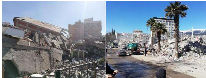
Figure 14. Complete destruction in Kahramanmaras city center (courtesy of the EEAT) [19]
