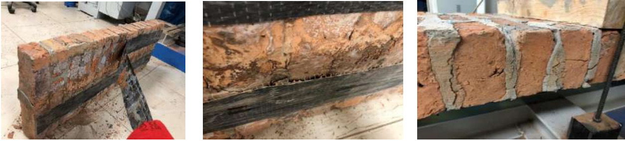
Fig 10. Failure mode of S-S2-L1 [31]
