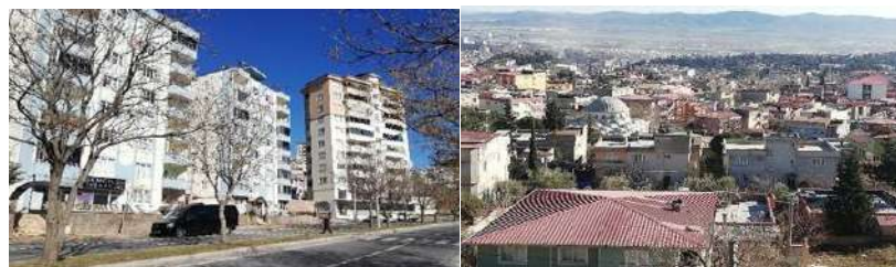
Figure 16. Buildings on the hillside of Kahramanmaras city center; a) (left) new high-rise RC frame buildings with no/slight damage, b) (right) old and low-rise RC and masonry buildings that performed relatively well during the earthquakes (courtesy of the EEAT) [19]
