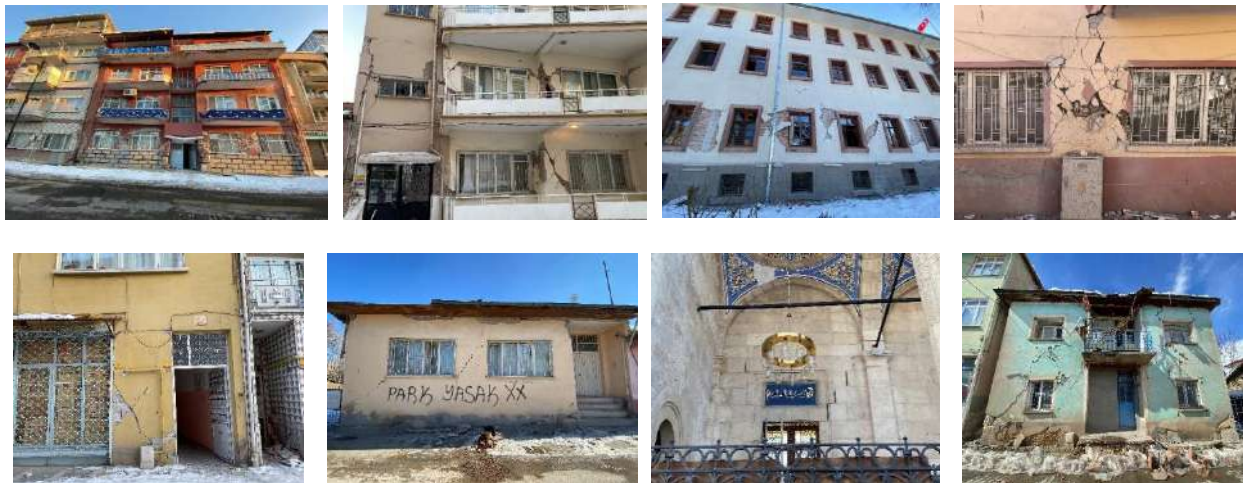
Figure 13. In-plane damages in masonry structures in Malatya [10]
