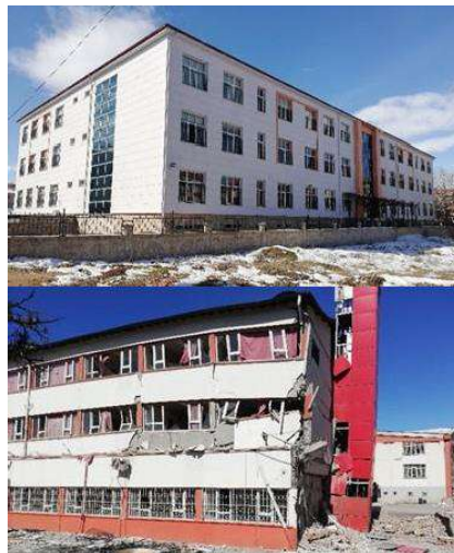
Figure 18. a) A school building with no damage in Golbasi (Adiyaman), (top) b) a severely damaged school building in Kahramanmaraş city center (bottom) (courtesy of the EEAT) [19]
