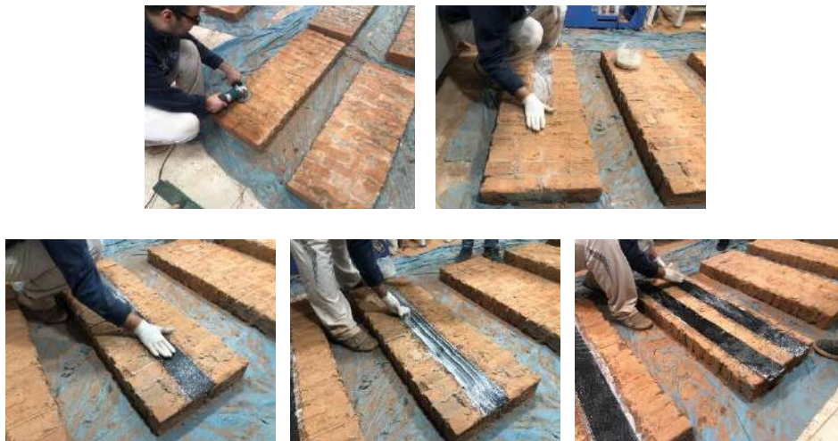
Figure 5. Strengthening processes of masonry panels [30]
