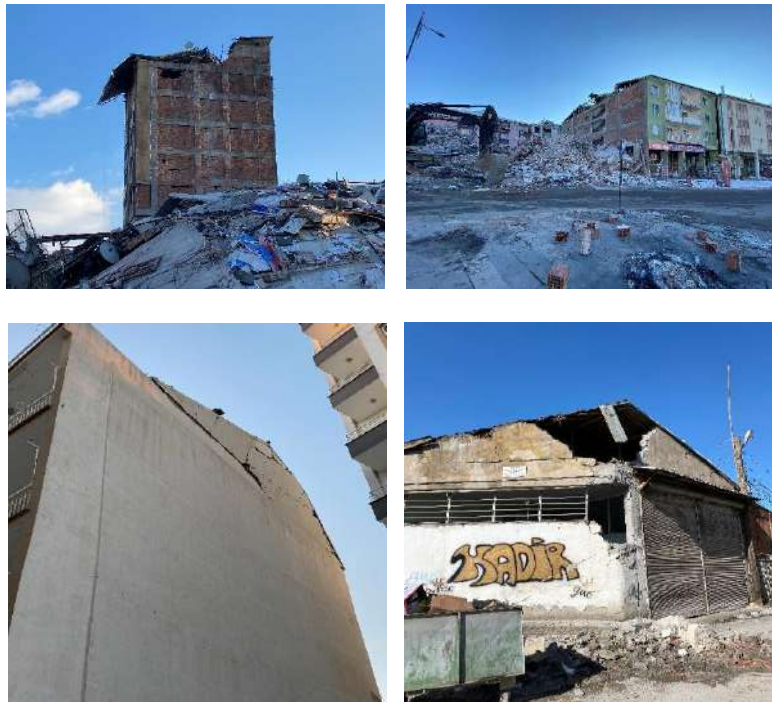
Figure 8. Failures of gable walls in Malatya [10]
