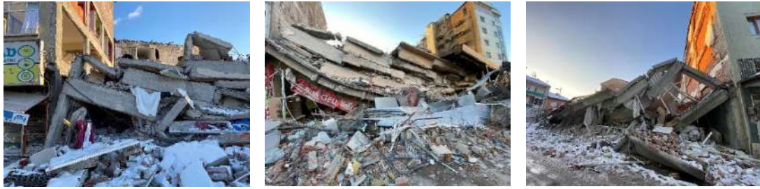
Figure 9. Failures due to strong beam- weak column combination [10]
