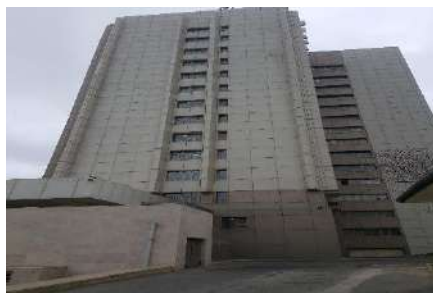
Figure 3. Northern facade of the educational building of the Azerbaijan University of Architecture and Construction [5]
