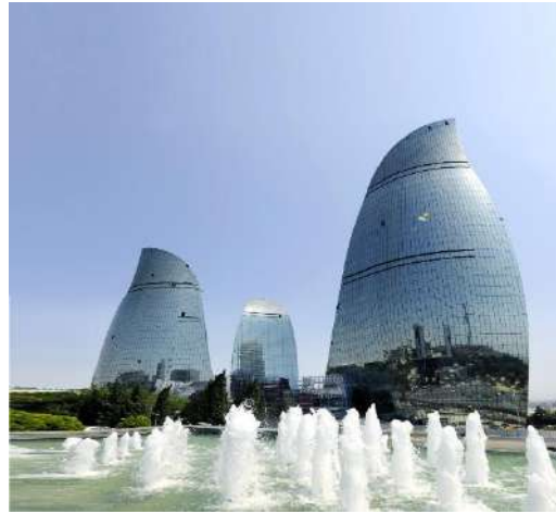
Figure 1. General view of the building from different directions [2,3]
