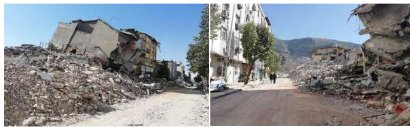
Figure 12. The photos of total destruction in Antakya, Hatay (courtesy of the EEAT) Antakya city was recognized for its cultural diversity and richness and it resided many historical structures, including invaluable heritage belonging to different religions. Unfortunately, most of these structures were either severely damaged or collapsed during the sequential earthquakes of February 2023 in Turkiye (Fig.13) [19]
