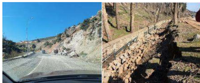
Figure 8. a) Rockfall on the road route around Nurdagi, b) damages due to lateral spreading along the stream channel in the Fevzipasa neighborhood of Islahiye [19]
