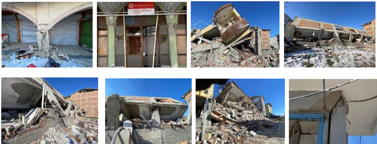
Figure 10. Damages caused by inadequate reinforcement [10]
